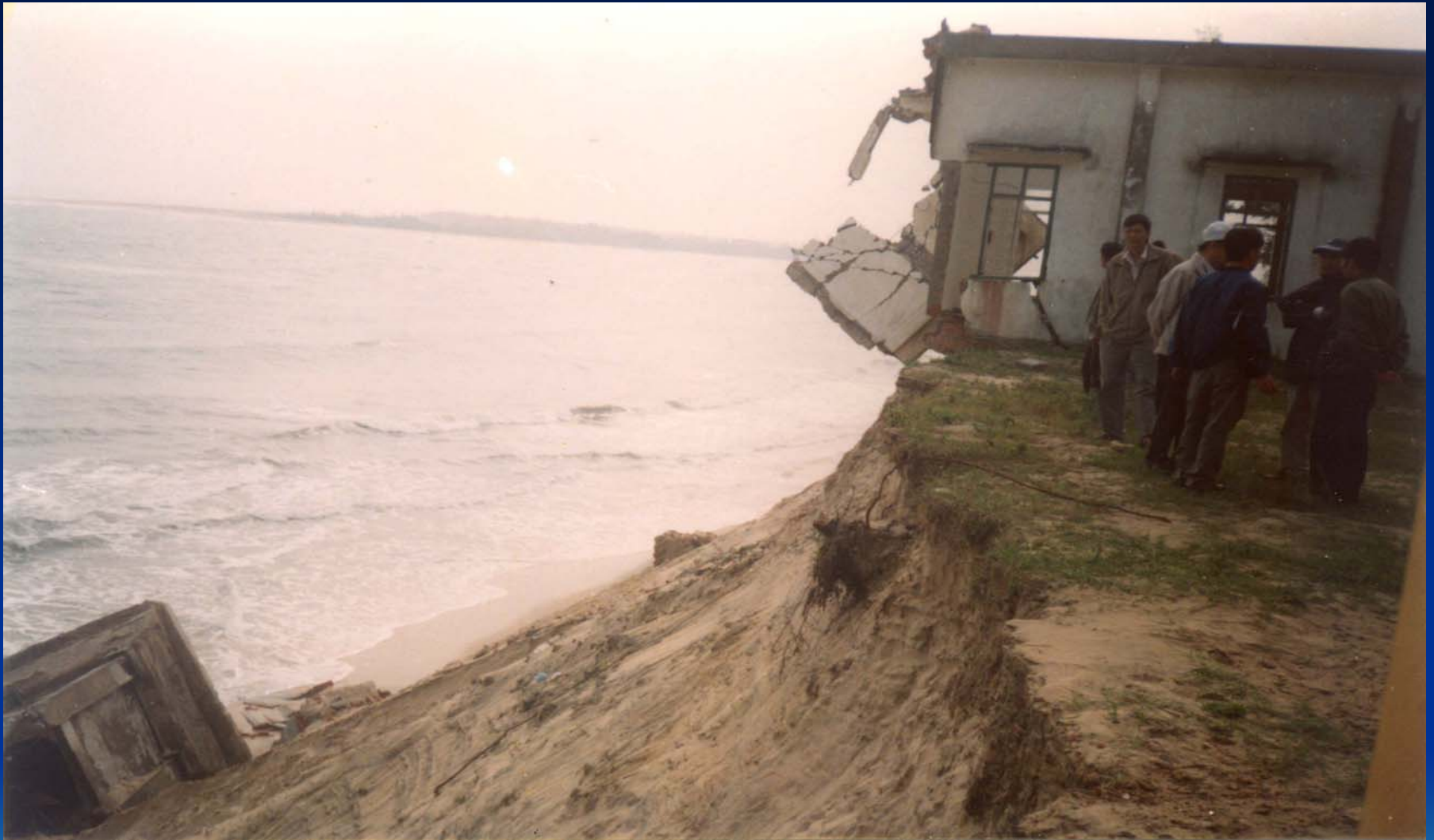
Picture 2. Landslide in Thuan An mouth
