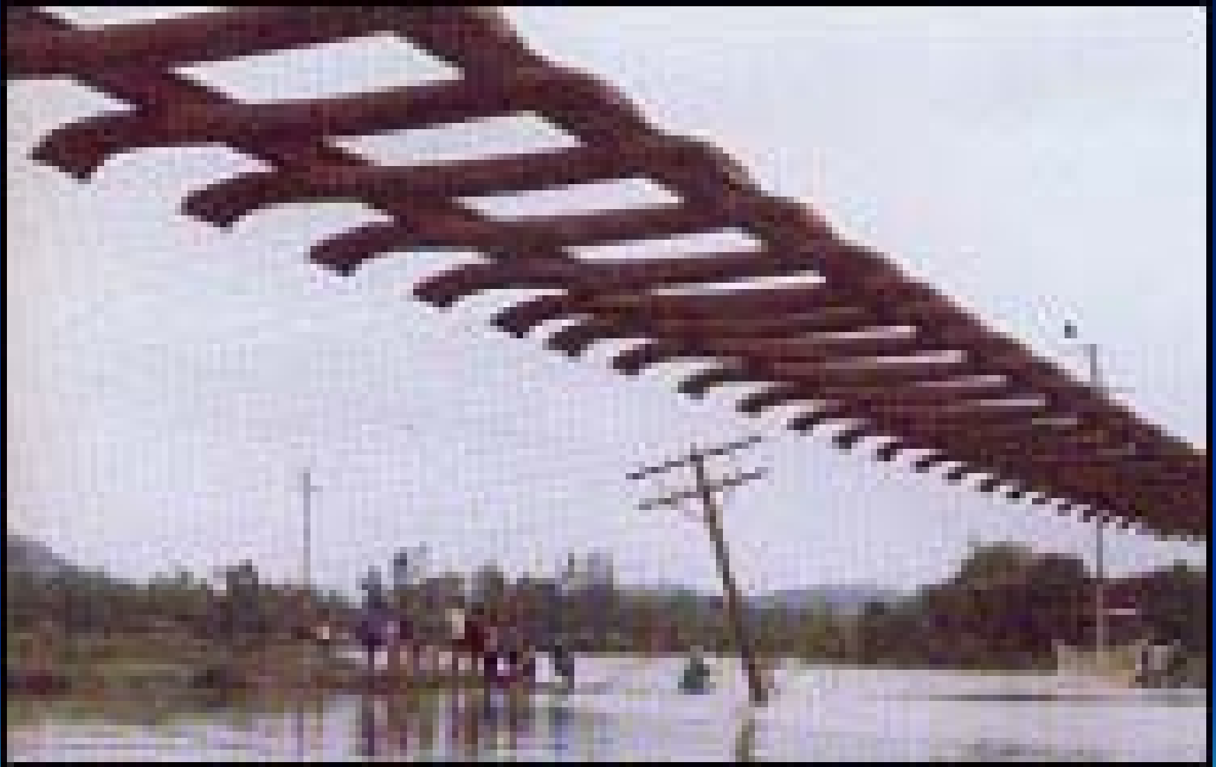
Picture 1. Railway after flash flood in Cong Bac - Thua Thien Hue (1999)
