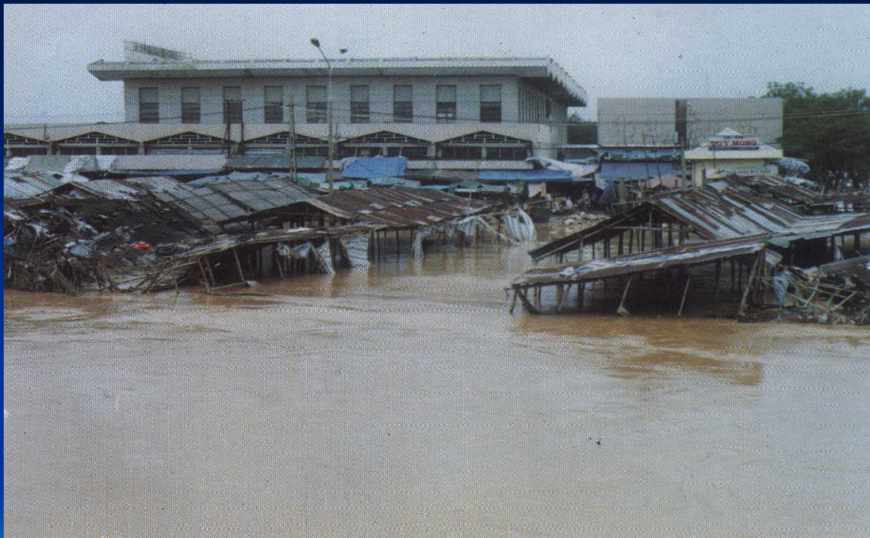
Picture 4. Flooding in Dong Ba market Nov, 2004
